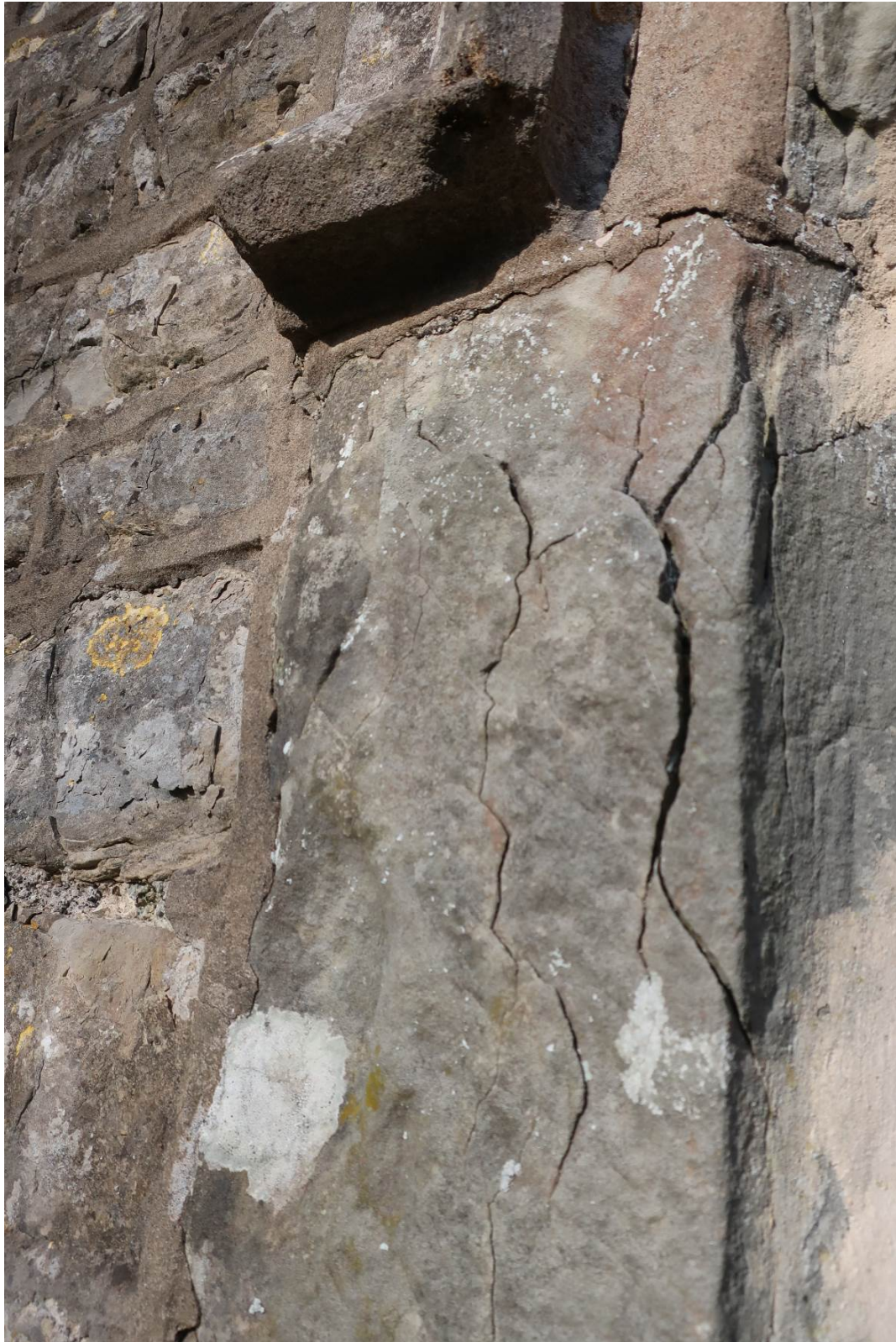
Figure 5 Delamination of the left-hand side the sandstone and lichen colonisation on the surface
