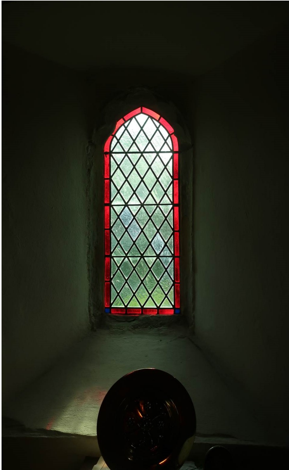
Figure 2 Photo taken from inside the chancel showing that there is no visible damage to the indoor wall of the window
