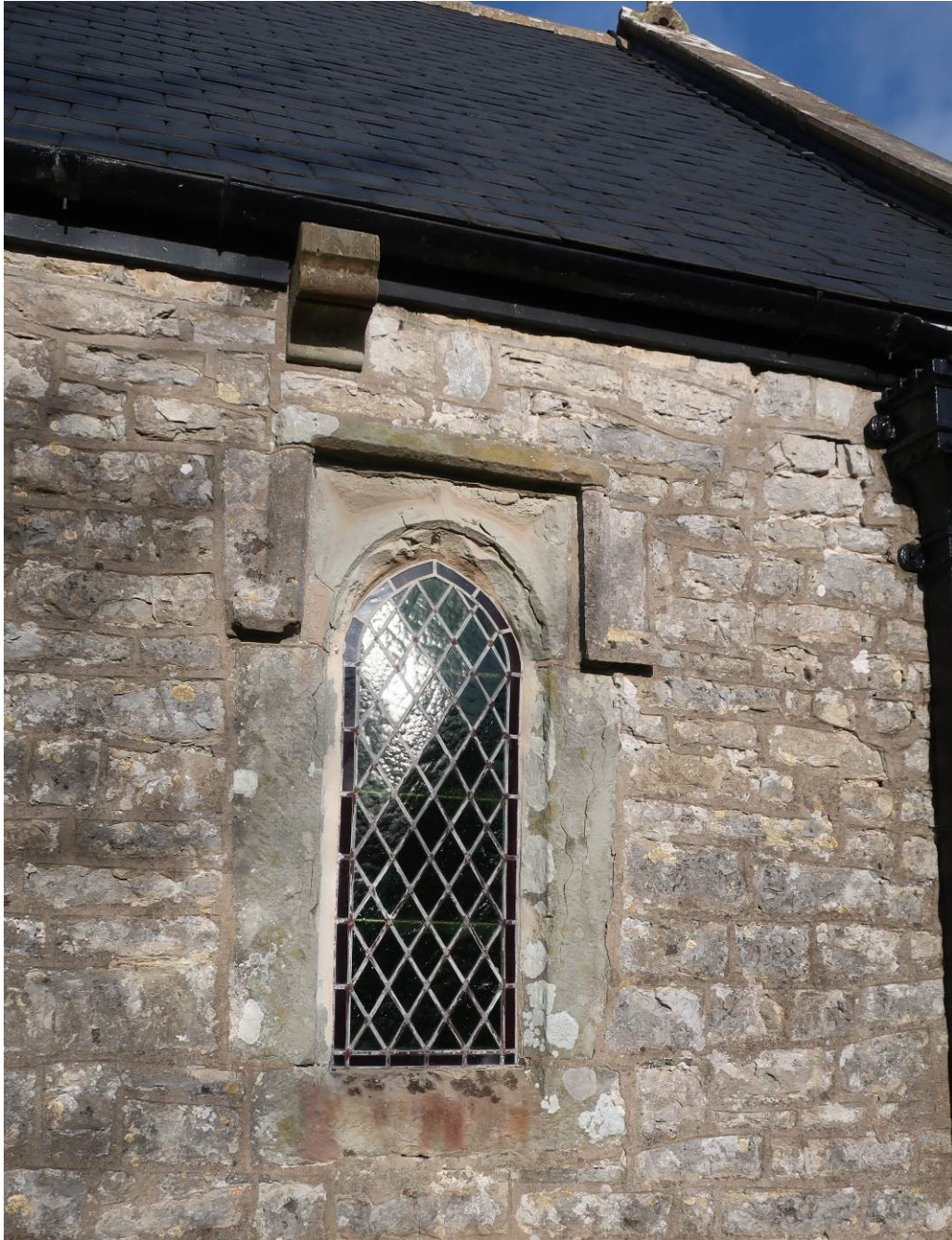
Figure 1 Picture taken from ground level of the current state of the chancel window and on the top and right-hand side there is evidence of the French draining system
