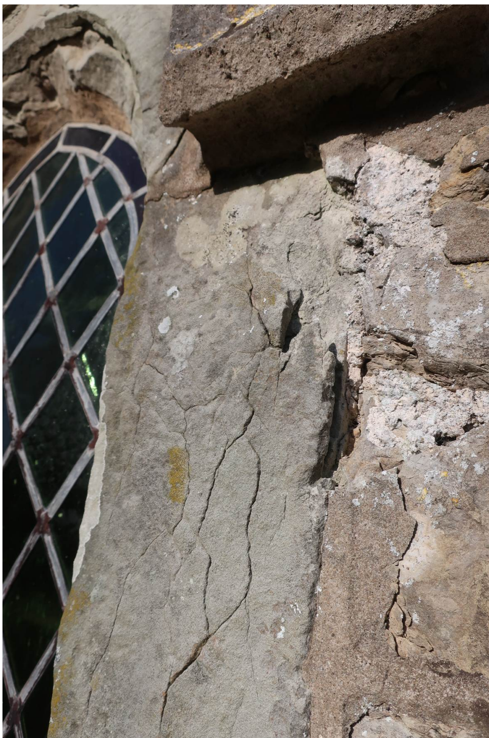
Figure 6 Severe delamination of the right-hand side sandstone leading to loss of stone surface
