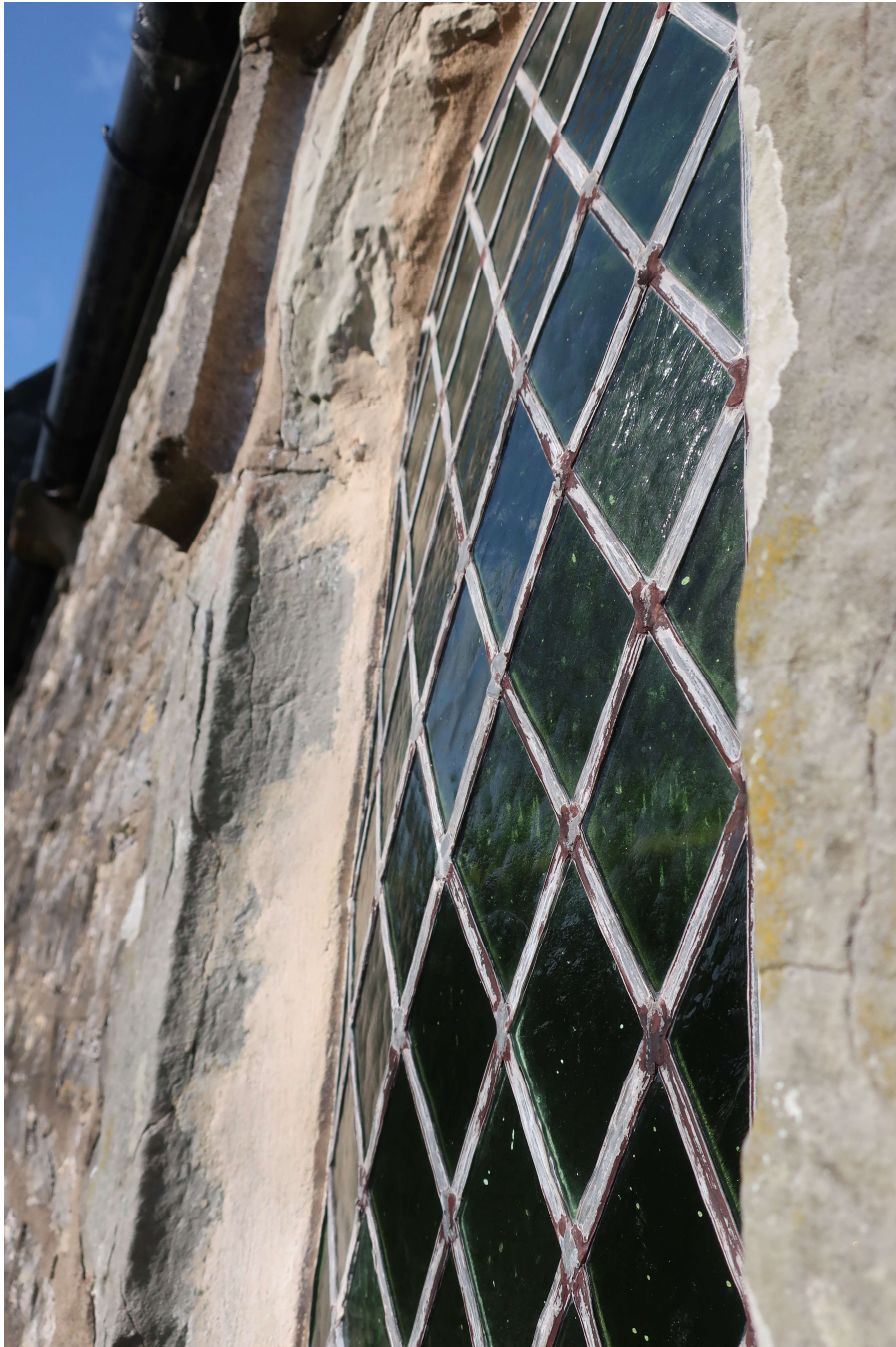
Figure 7 Side photo showing the bulging window
