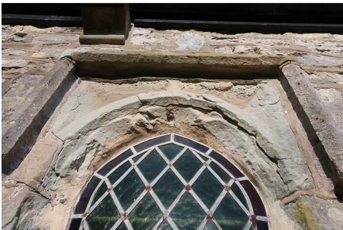
Figure 4 Close up on the arch and hood moulding structural damages caused by the delaminated stonework and incorrect hard cement pointing
